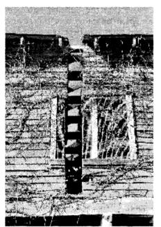
**Figure 4** Dissection cut through the building leaving structural members intact.
